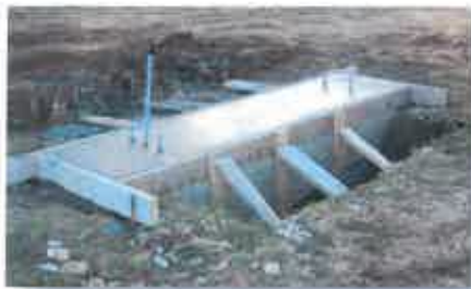
The old sign is out and the new base is poured
